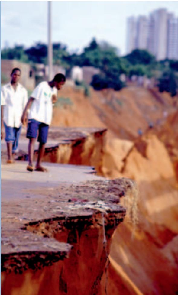
Figure 8: The main street in Maputo has been eroded and washed away due to long lasting rainfalls and inundations, Mozambique
